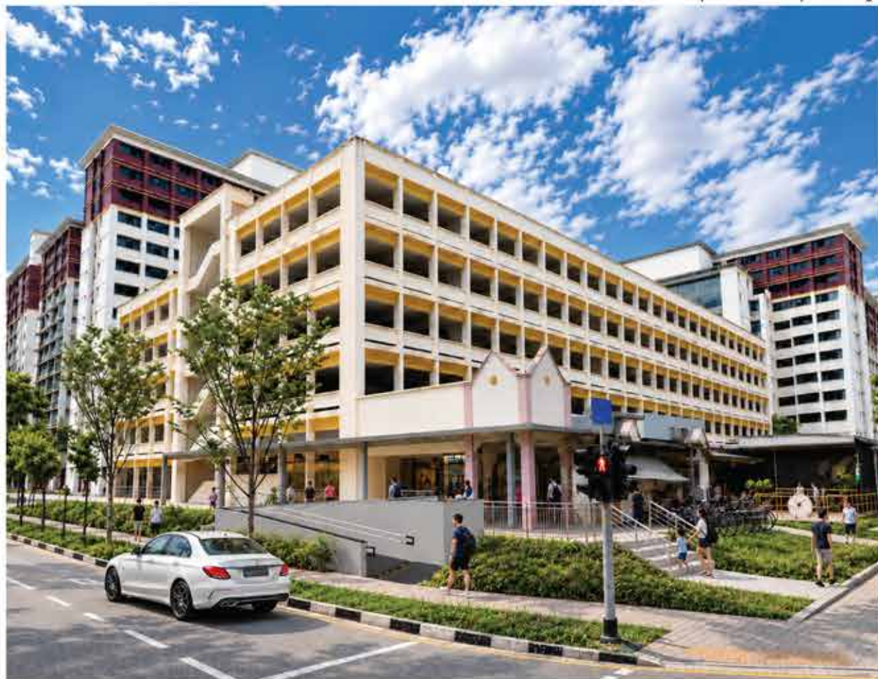
UPGRADING OF PRECINCT PAVILION FINISHES
