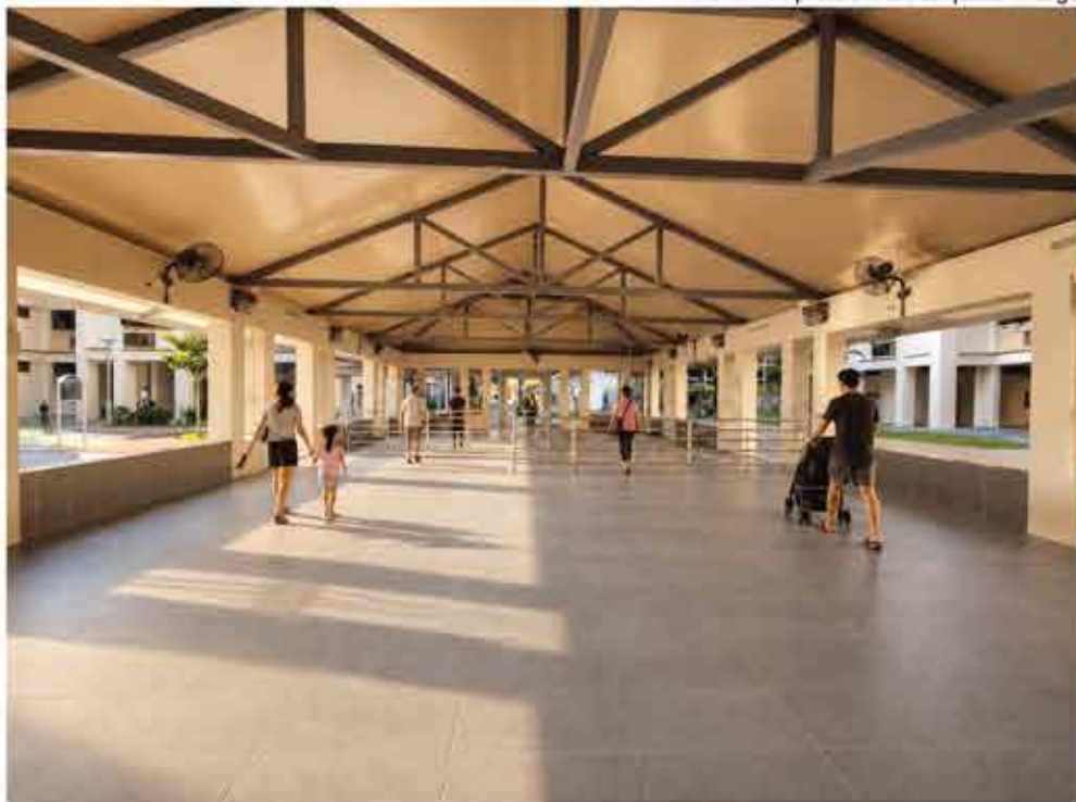
UPGRADING OF PRECINCT PAVILION FINISHES
