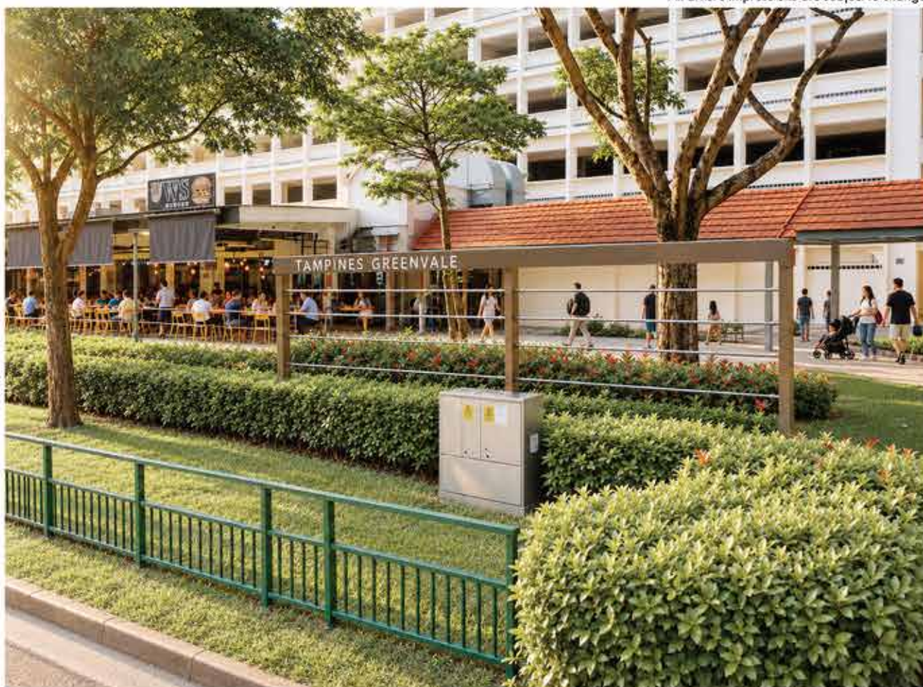
UPGRADING OF PRECINCT PAVILION FINISHES
